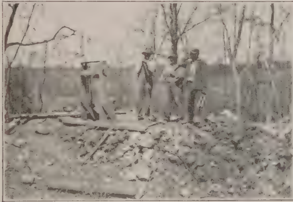
(33) Operating prospect shaft with hand windlass. Breaking ground on Jones vein. Holly Ore and Mining Co.
